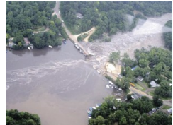
Figure : A dam break
